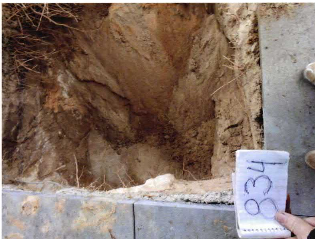
Picture 2: UST 834Azalea excavation.
